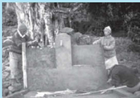
Nepali villagers install a community water tap
